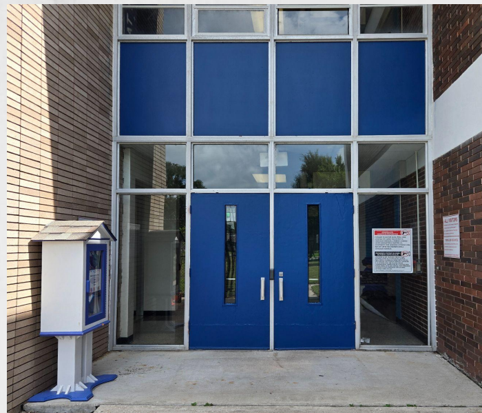
Doors facing Groveswood
